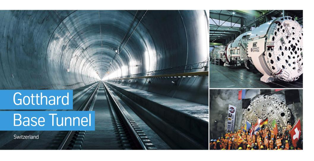
Since June 2016, the Gotthard Base Tunnel connects the two Switzer cities Erstfeld and Bodio. With a length of 57 kilometers, Switzerland unites northern and southern Europe by rail through the Alps. This once-in-acentury project is the longest railway tunnel in the world and consists of two single-track tunnels. The Gotthard
